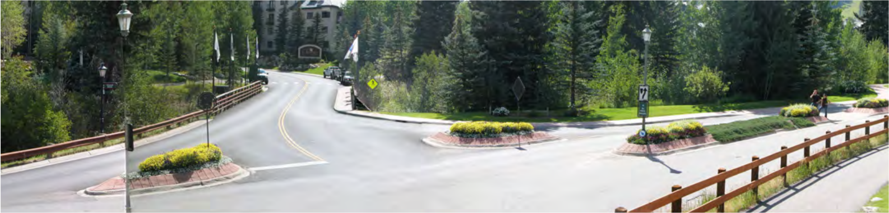
EXISTING CONDITIONS AT VILLAGE ROAD AND OFFERSON ROAD INTERSECTION
