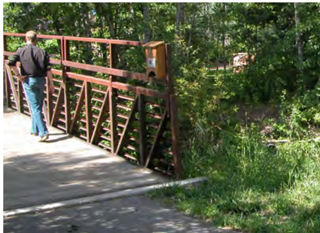
BEFORE VEHICULAR-USE BRIDGE
