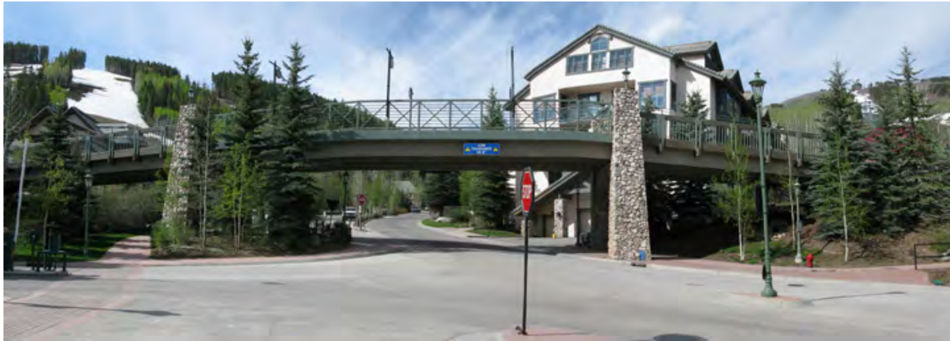
EXISTING BRIDGE AT VILLAGE CORE ENTRANCE
